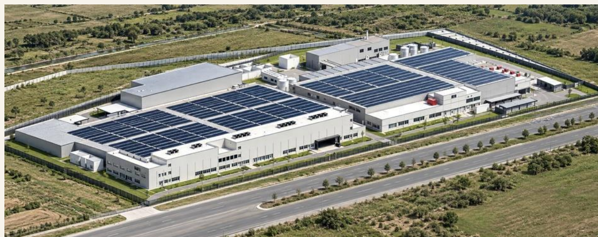
Rooftop solar, Ninh Thuận
