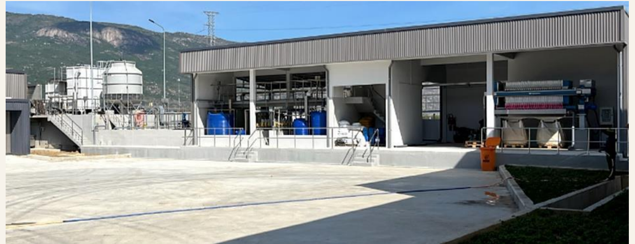
Wastewater treatment, Ninh Thuận
